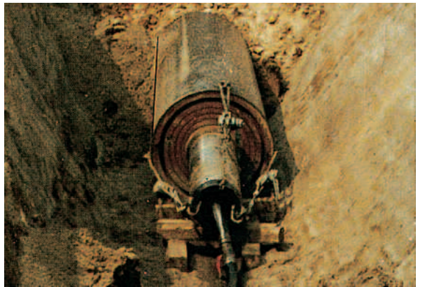
1200 mm pipe being driven 22 mtrs.
