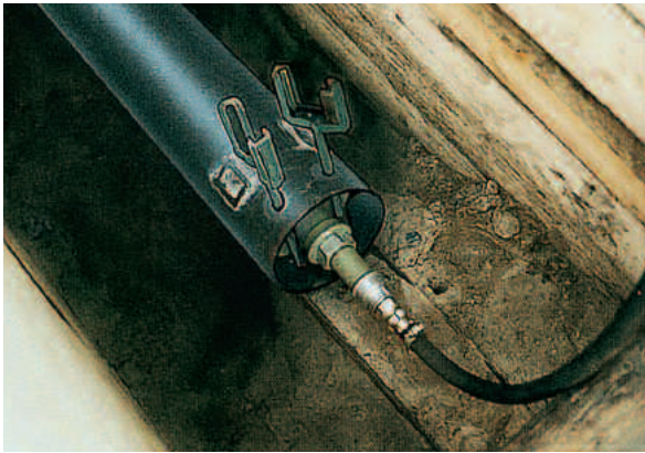
Installing cleaning element.
