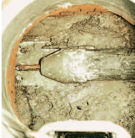
IPM 155 with PVC end seen from manhole.
