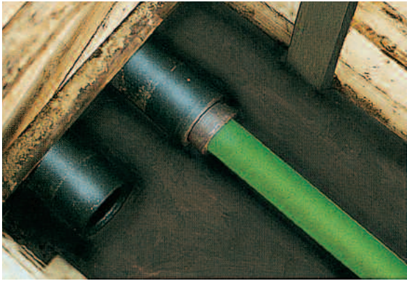
250 mm steel pipe 24 mtrs. under embankment.
